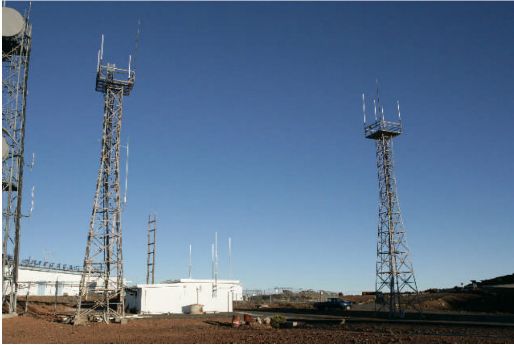
FIGURE 1-5 Two Existing FAA RCAG Towers
